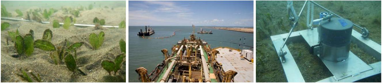
Dredged material from ports is saline and therefore is unsuitable for agricultural and vegetation rehabilitation uses. Establishing any vegetation on spread or stockpiled dredged material is expensive and can take years to become successful. Moving the material from a land based site would involve large numbers of truck movements considering the volumes involved creating community amenity issues and increased greenhouse gas emissions.
